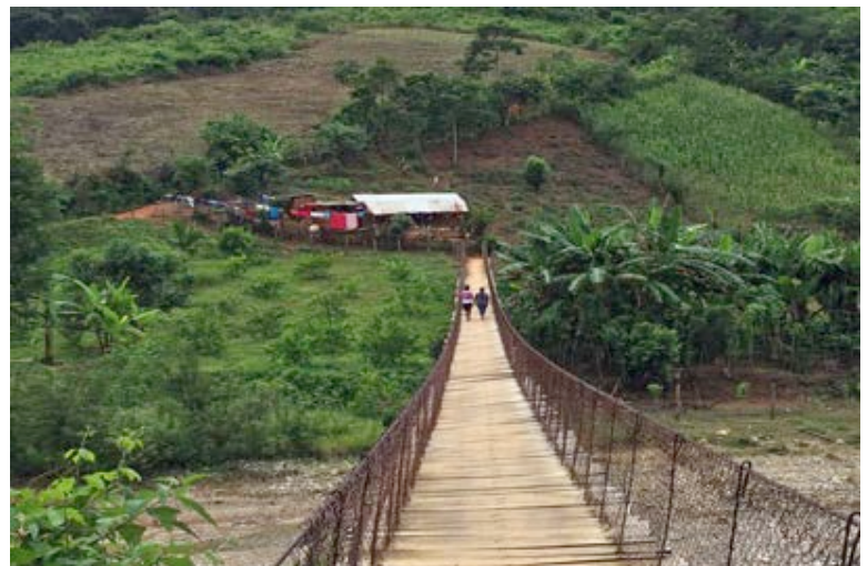
Footbridge in a remote Chiapas community
